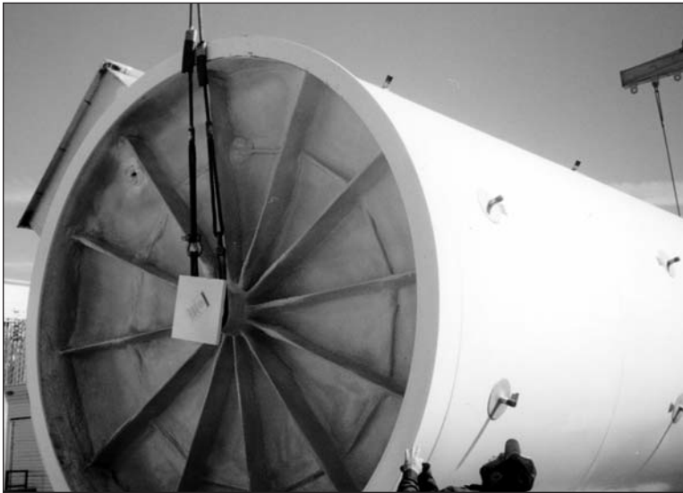
Figure 7 - Lifting the Silo from the Trailer and Erecting
