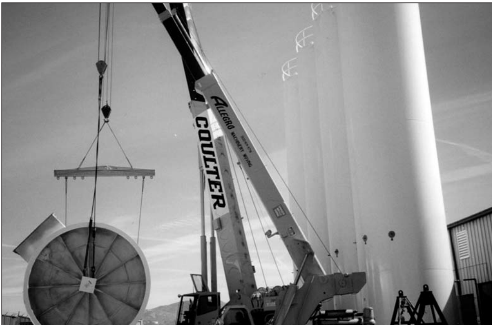
Figure 5 - Using a Spreader Bar to Lift the Silo from the Trailer
